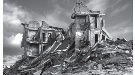
COLLAPSE (P. 29, Act. 2)
